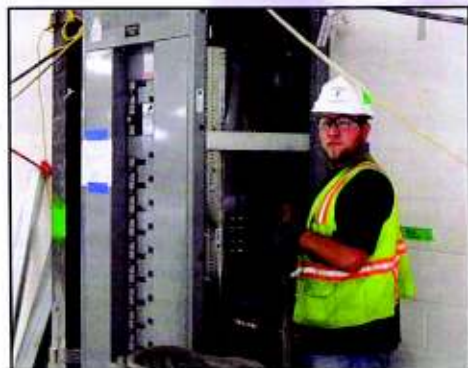
Apprentice Ethan Frank at the Solyndra project for Sprig Electric
