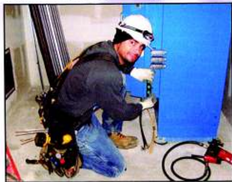
Apprentice Michael Cotroneo at the Altenheim project in Oakland
