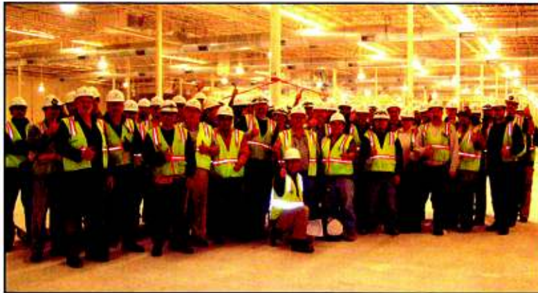
Local 595 members working for Sprig Electric at one of the Solyndra sites in Fremont. Another site is also underway with Rosendin Electric.
