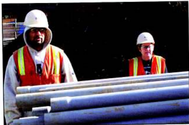
Apprentice Gagan Bahad and JW Cynthia Montero at the Washington Hospital project in Fremont
